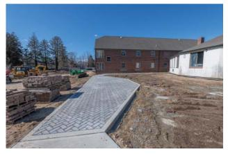
A permeable paving system will aid in rainwater drainage and connect the library with parking lots and outdoor program areas.
